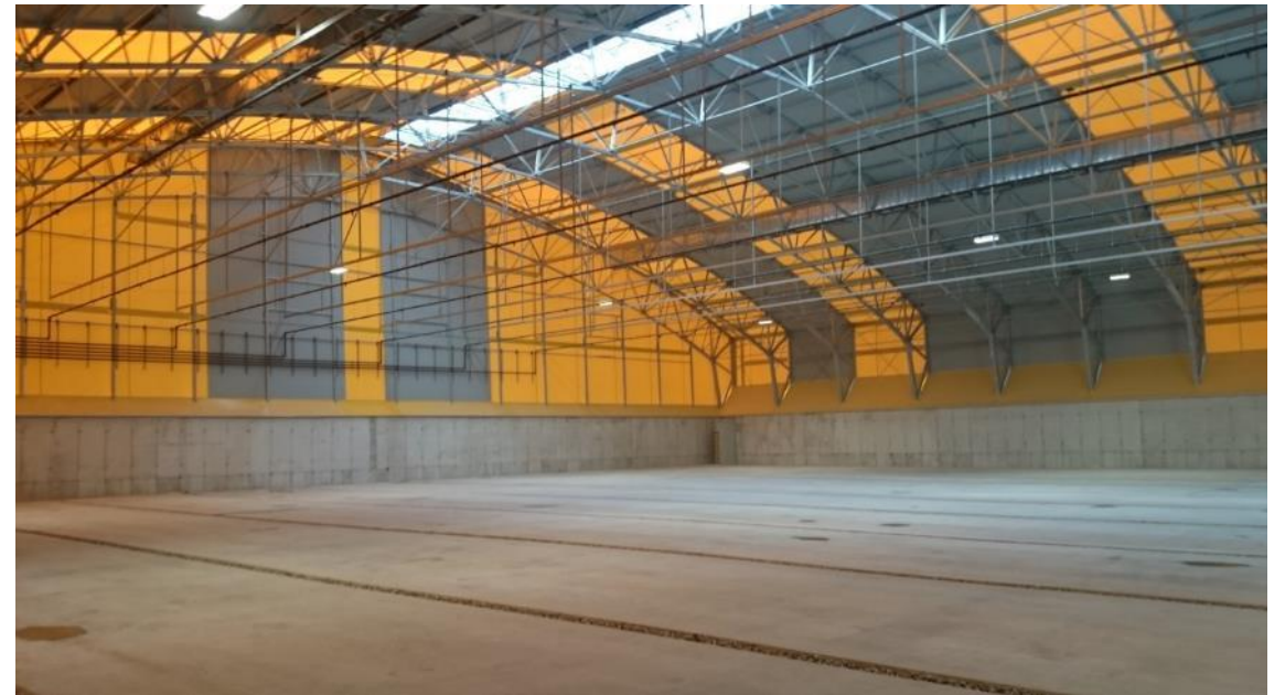
Waste management centre, Slovenia 53x81,2 m
