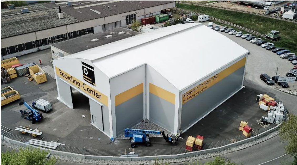
Recycling centre, Switzerland 29,8x36,1 m
