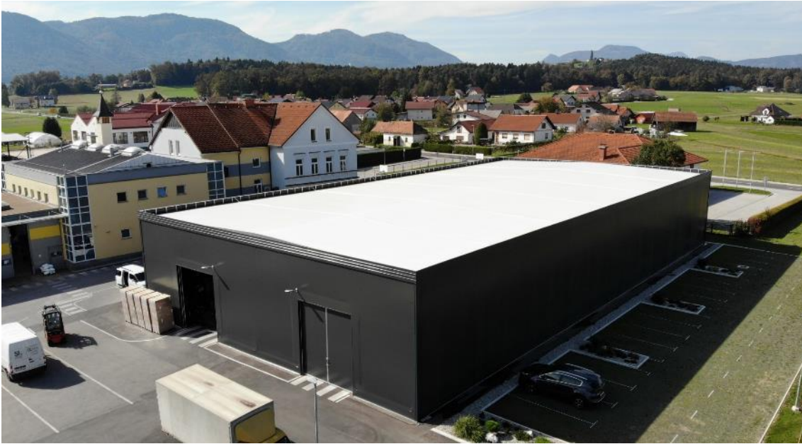
Warehouse, Slovenia 25x48 m
