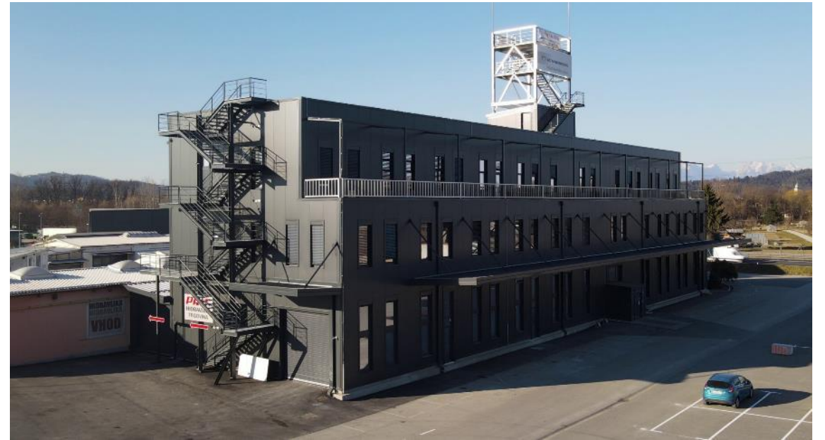
Multipurpose business facility, Slovenia 15x55x9 m
